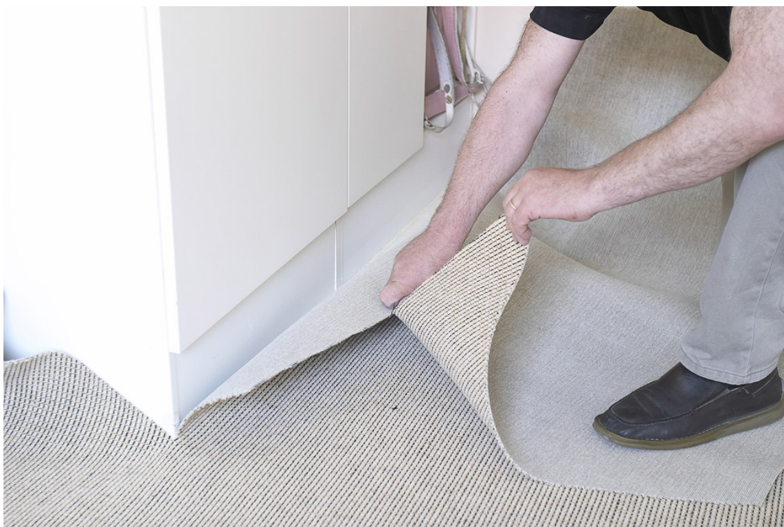
MARGIN: Grovtilpass teppet.
